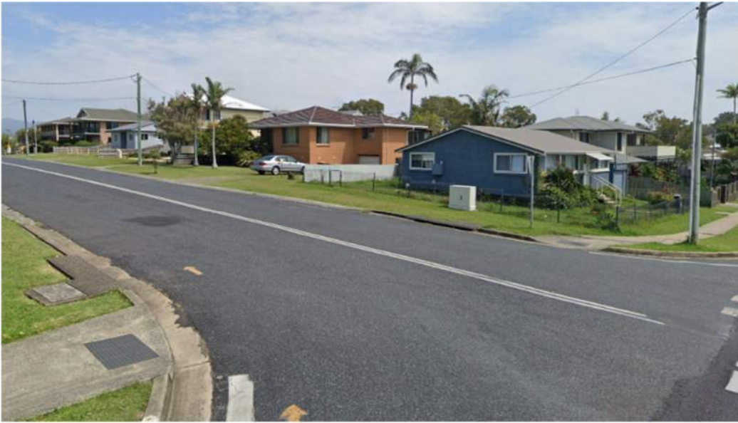
^ Crossing of Eighteenth Avenue at junction with First Avenue. New footpath required along northern side of Eighteenth Ave (right side of photo). To be co-ordinated with existing road signs and services. The existing kerb ramp and part of footpath on First Ave may need to be re-built to allow the new footpath to join in a compliant manner.
